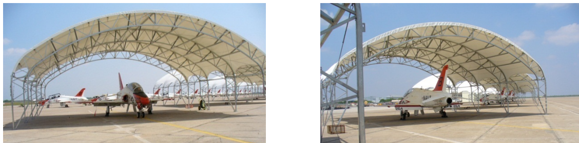
Figure 4-1 Examples of Weather Covering
