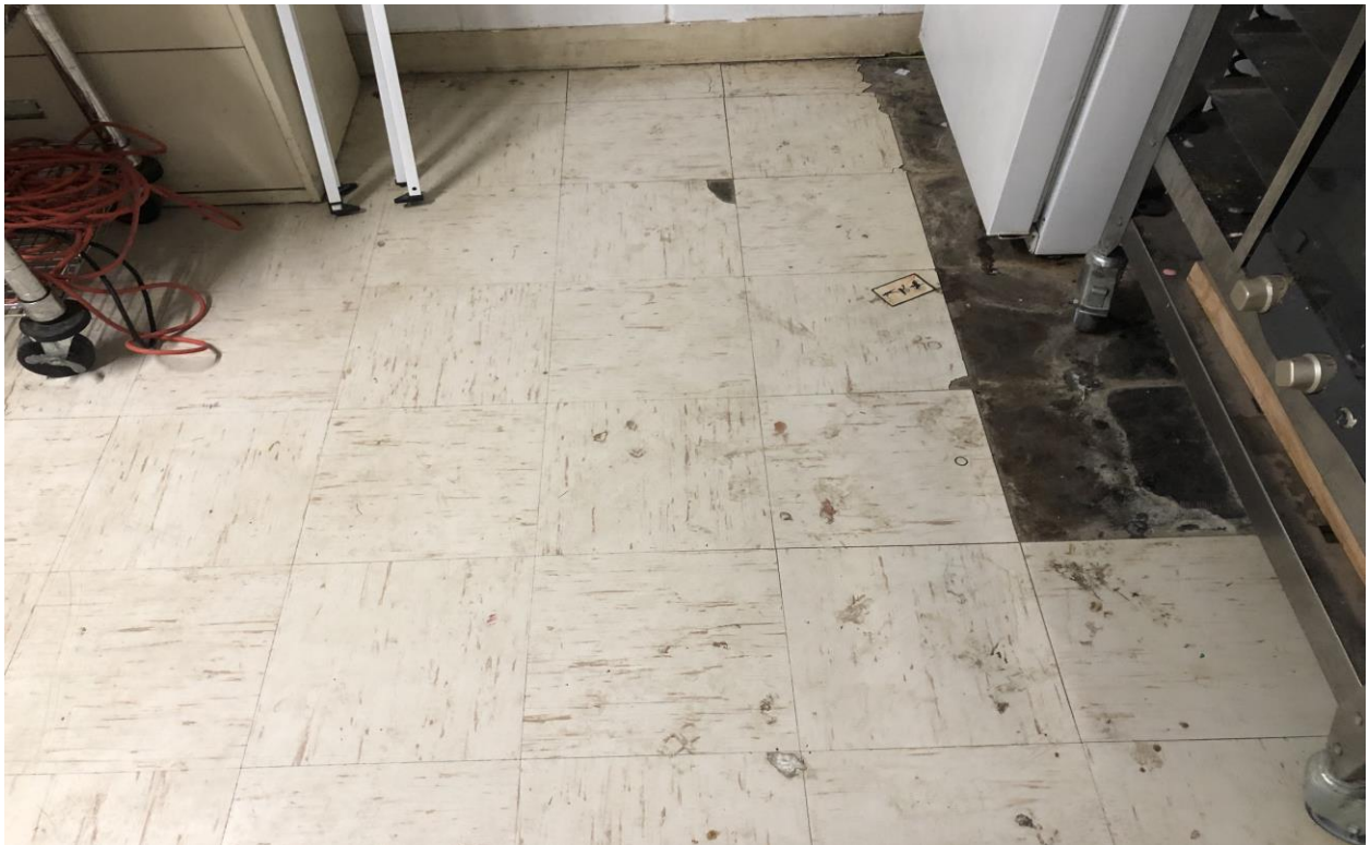
Hanger Building 1 st Floor: Kitchen area with visible Black Mastic
