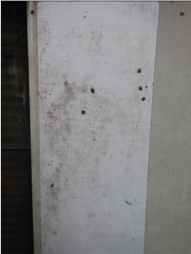
7.3 Item 1(Picture) The data plate for the condensing unit. Mfg 2002
