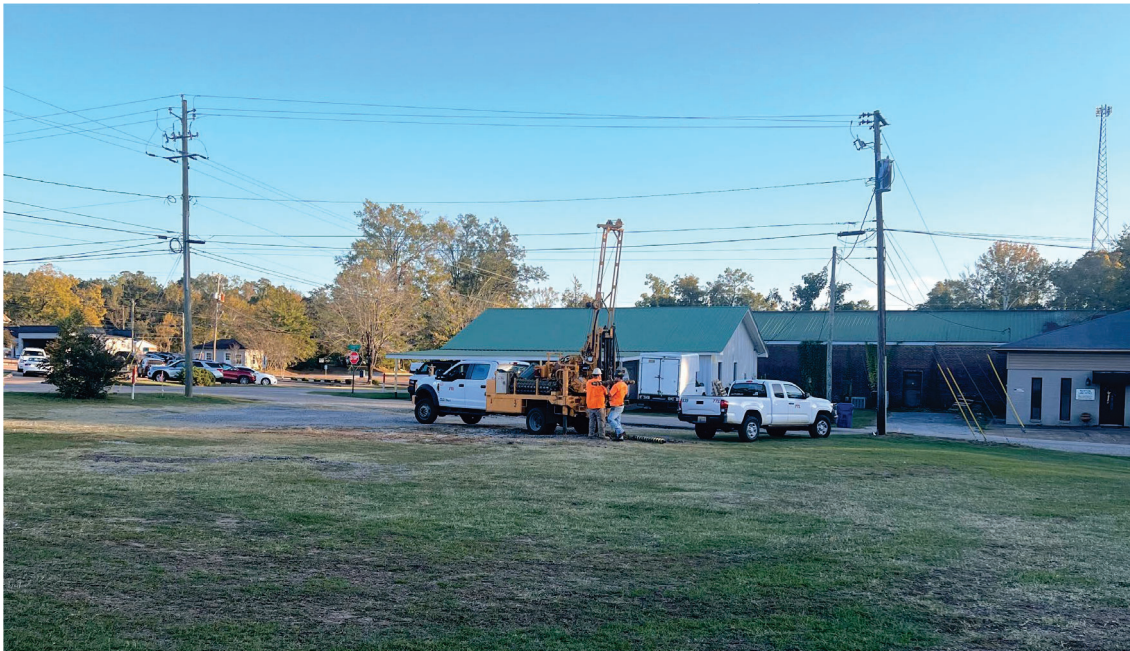
This photo is facing south across the site and shows boring B-08 in the process of being drilled.
