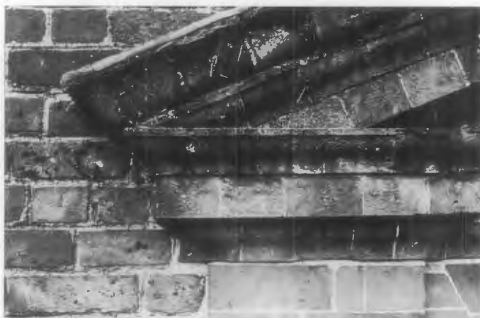
Figure 19. Mortar joints of 18th century brick buildings were often as much as 1/2 inch wide, cut flush and struck with a grapevine joint, but for window and door surrounds where a finer quality rubbed brick was used, mortar joints were very thin. Photo: National Park Service Files.
